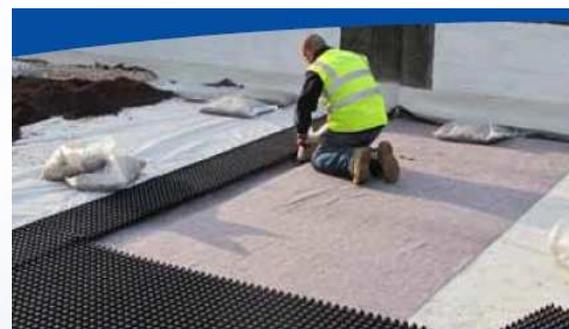
Above: Biodiverse roof installation showing the root barrier, drainage board and filter fabric
